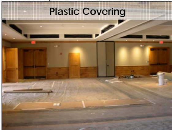
Proper Carpet Protection Kraft Paper and Masonite
