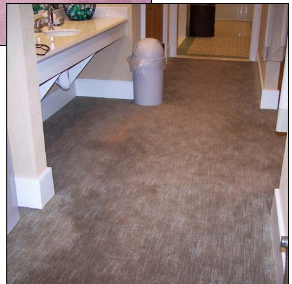
Shading & Highlighting – Locker Room
