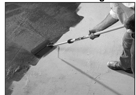
Rolled Application of Curing Compound
