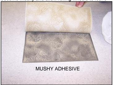
marks in the flooring material that make the surface look like there was an off road rally that took place on the floor. Since welded seam sheet goods are not permeable, moisture in the substrate can soften adhesive, allowing the flooring material to release and become more easily susceptible to indentations.
